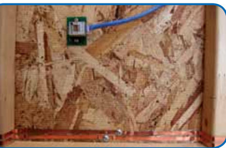
Wall Moisture Detection System
