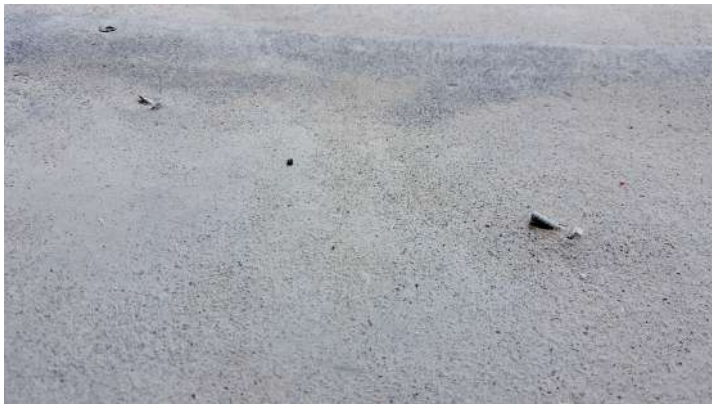
At the Parq site, we found nails and screws literally embedded into the membrane
