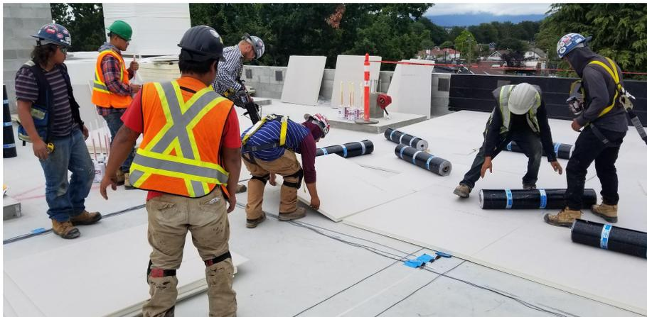
*Above: FutureCast's sensor grid sits on the lowest layer of a conventional roof assembly*
