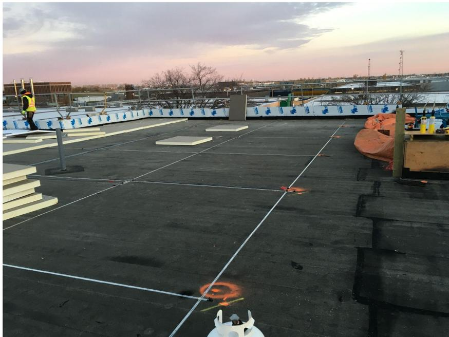
*Above: FutureCast sensor grid comprises MDS tape laid out in a grid*
