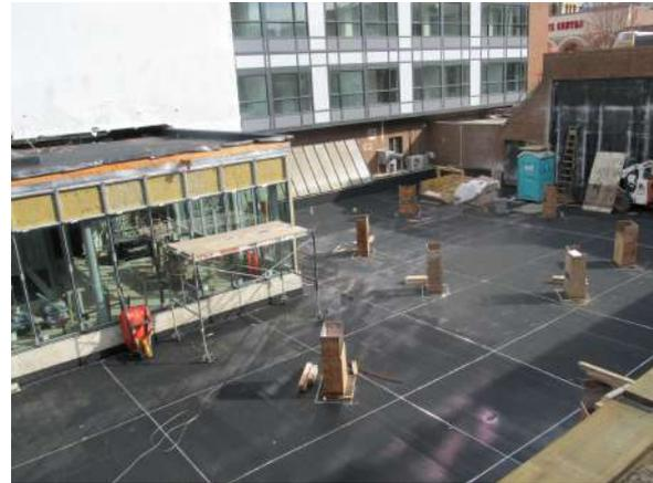
■ FutureCast sensors installed in a grid on top of a roof membrane before overburden
