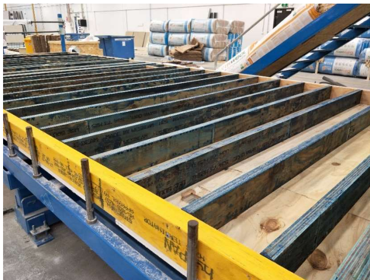
Figure 2: LVL wall frame on Strongbuild's wall line, Image Credit: Strongbuild
