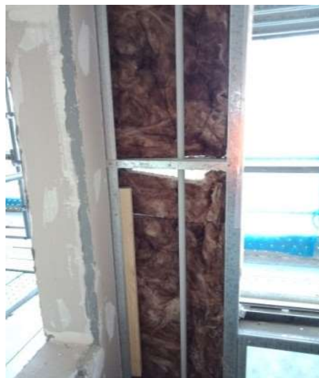
Figure 18: Wall cavity before the wall gets closed, Image Credit: TDA
