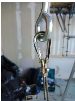
Figure 10: Connection Eye-bolt and stainless steel wire, Image Credit: TDA
