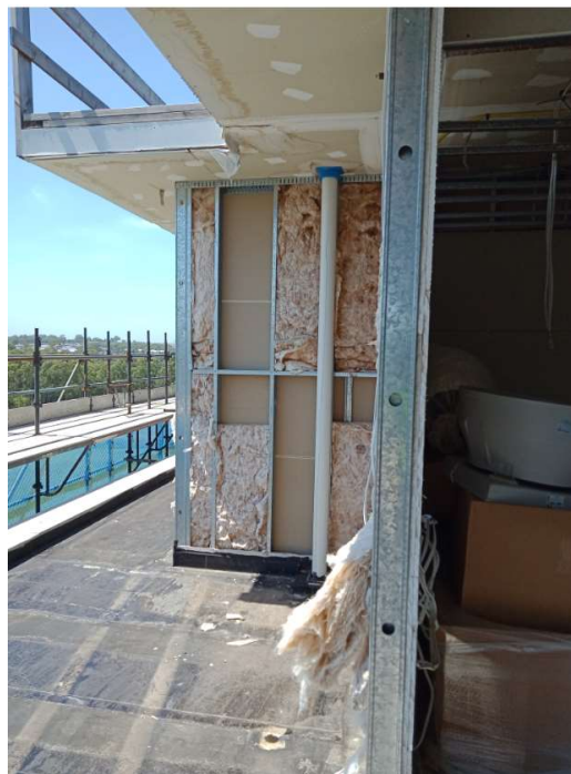
Figure 5: Exterior Steel Frame Walls, Image Credit: TDA
