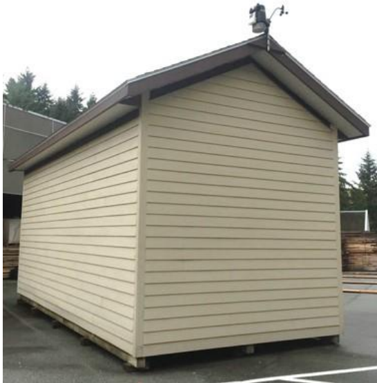
FIGURE 1: Exterior of the Finished Test Hut
